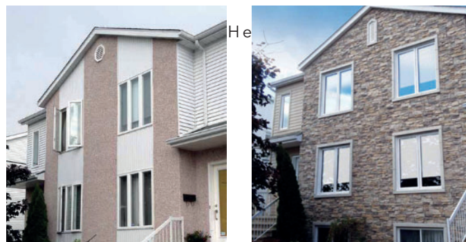
Fig. 7: Before and after - renovation with Beonstone panelized stone siding.
